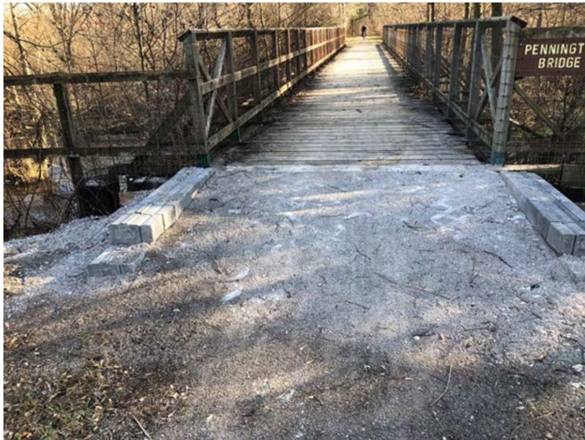
Pictured: New bridge ramp on Pennington Bridge
